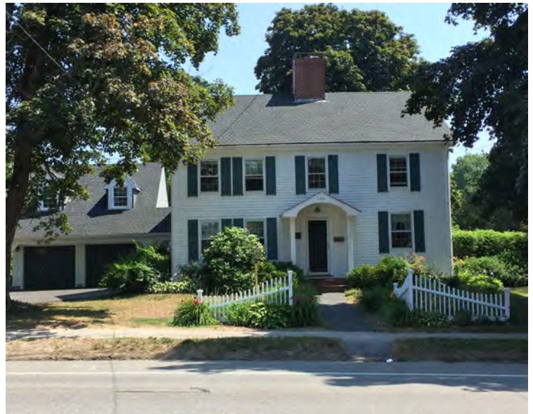
HATEVIL HALL HOUSE, c. 1762 111 Hillside Road, Falmouth
